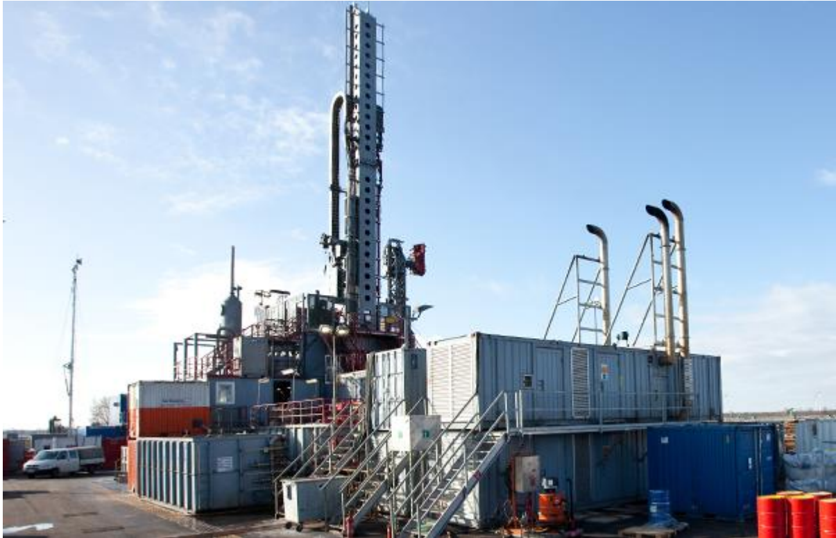
Figure 9.3: Photo of DrillTec VDD 370 rig
