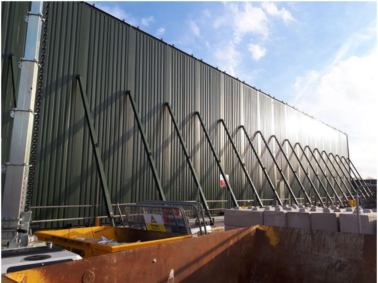
Figure 6.6: Example demountable acoustic barrier
