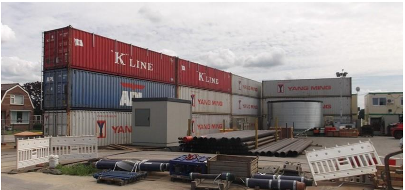
Figure 6.7: Example barrier constructed from containers
